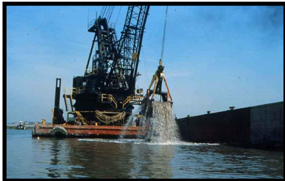
Figure 5-5. Mechanical dredge (clamshell bucket and barge).
