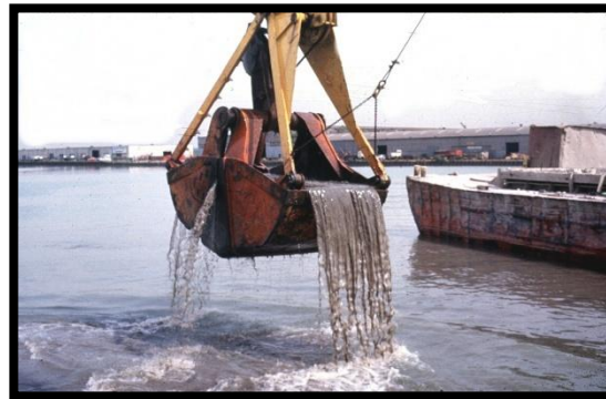
Figure 5-5. Mechanical dredge (clamshell bucket and barge).
