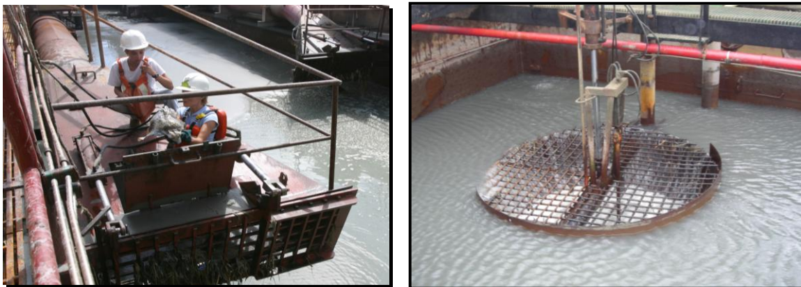
Figure 8-14. Photographs of hopper dredge inflow (left) and overflow (right) screening.
